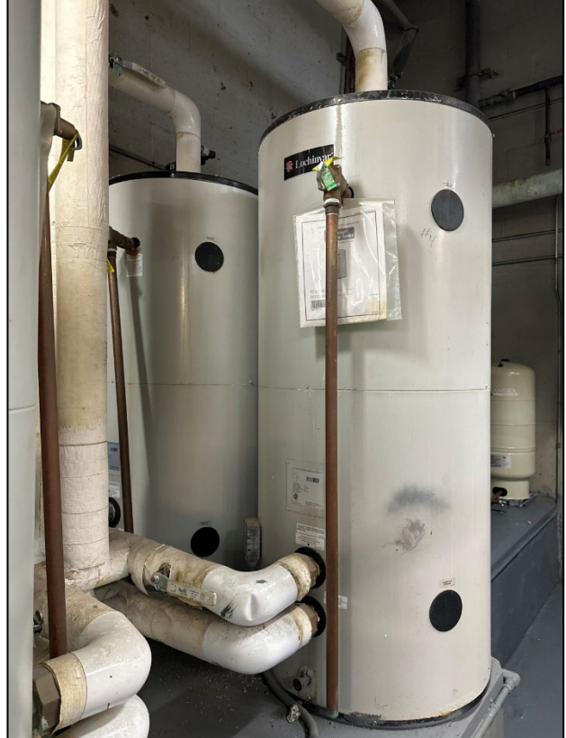
Existing Water Heaters, Storage Tanks & Piping
