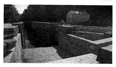
Scope of Work-Historic Restoration of the East Lock 2 Tenders House Wharton, NJ Concrete vault reconstruction included slabs and pedestrian bridge foundation. Natural stone walls demolition and rebuild both sides.
